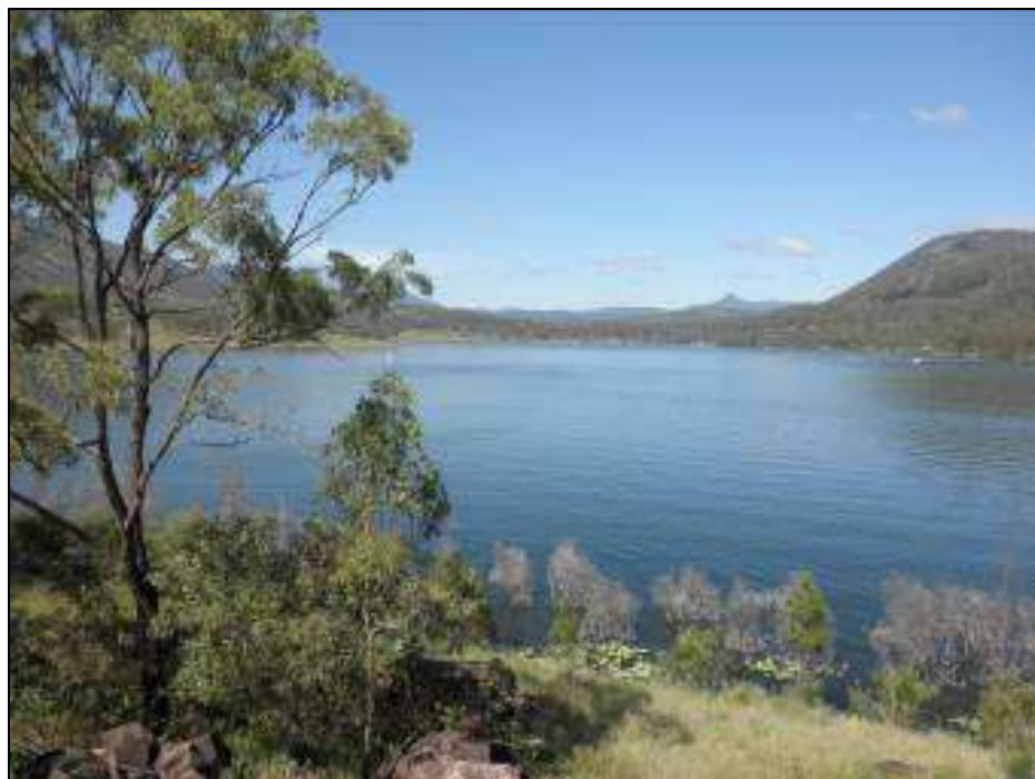
Figure 6: View of Lake from Spillway Entrance (looking south).
