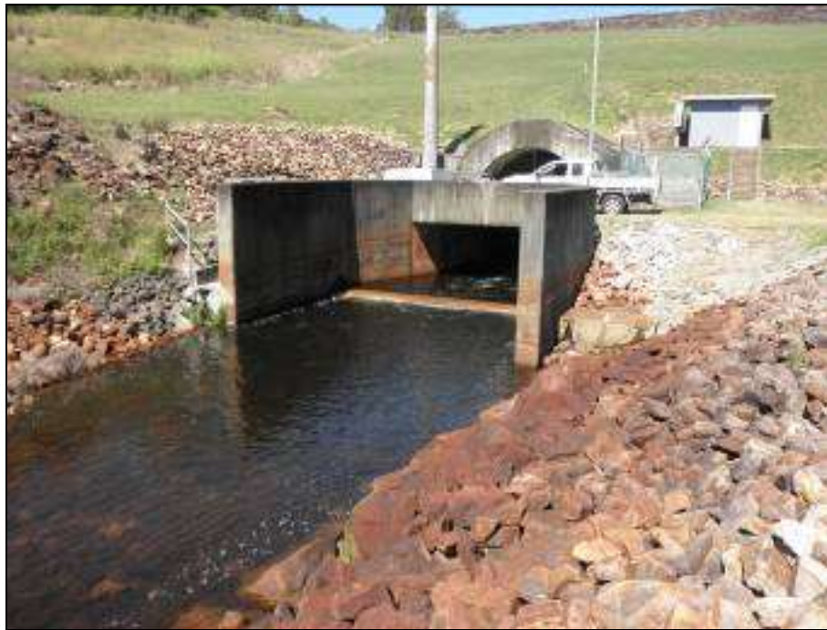
Figure 5: Maroon Dam Outlet – Discharge to Burnett Creek.
