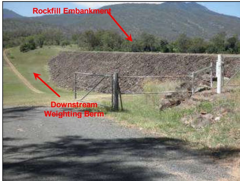
Figure 3: View of Downstream Embankment of Maroon Dam.
