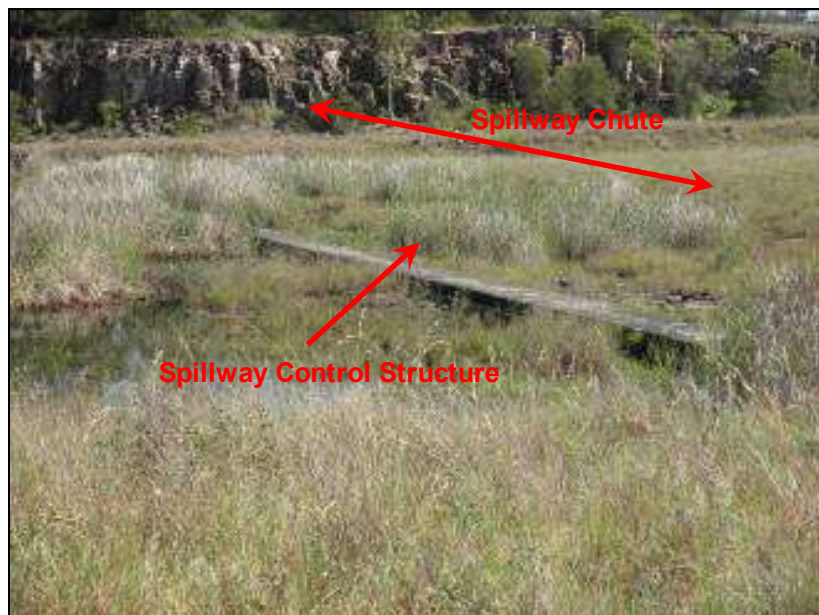
Figure 4: Maroon Dam Spillway.
