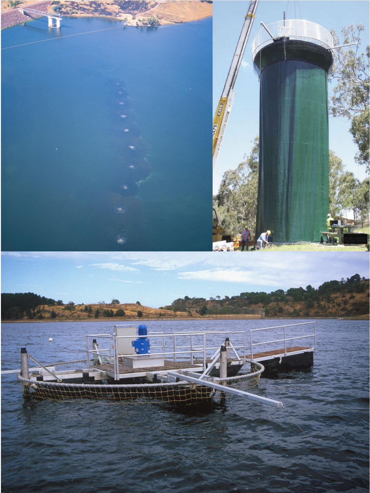
Figure 1. Destratification systems. Clockwise from top left: 10 bubble plumes at Chaffey Dam, NSW; WEARS draft-tube mixer awaiting deployment (photo courtesy WEARS); WEARS mixer deployed at Myponga Reservoir, SA.
