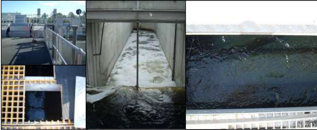
Figure 2. Sampling sites at the Oxley Creek Wastewater Treatment Plant.
