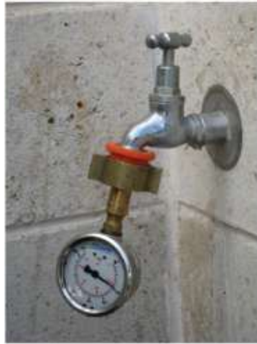
Figure 8: Pressure measurement at an external tap to confirm water flow from a rainwater tank.
