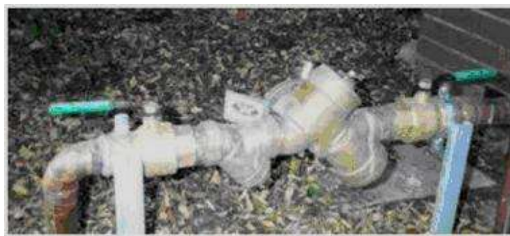
Figure 11: An example of a backflow prevention device. This prevents rainwater being drawn back into the potable mains supply in the event of a pressure drop in the mains water reticulation system.
