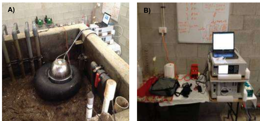
Figure 29: Example deployment of the gas analysis system in the field – A) The flux hood on top of the CDM MBR aeration tank; B) The gas analysis and data collection workstation.
