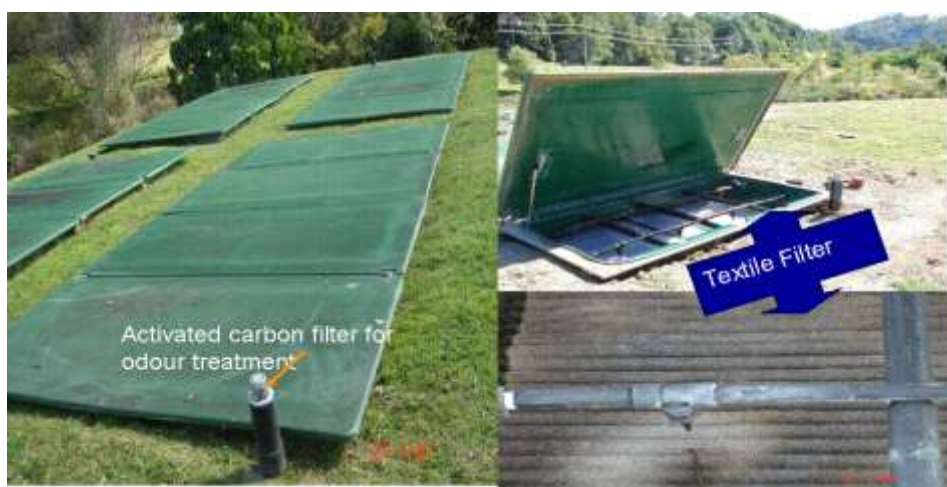
Figure 7: Photos of the textile filters in the Currumbin Ecovillage wastewater treatment and recycling plant.
