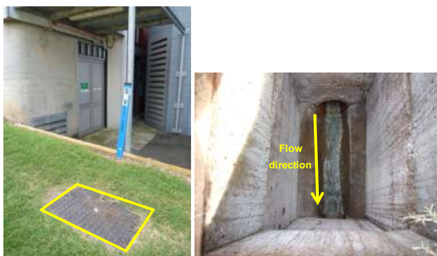
Figure 9. External and internal view of the selected manhole (0.8mx0.4mx1.0-1.3m) in front of Ipswich Hospital.
