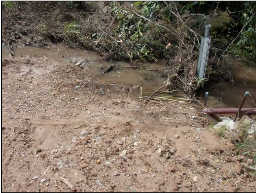
Figure 17: Sedimentation and erosion problem at Blunder Creek, Forest Lake due to civil construction subdivision works. The gauging station was relocated to suitable location.
