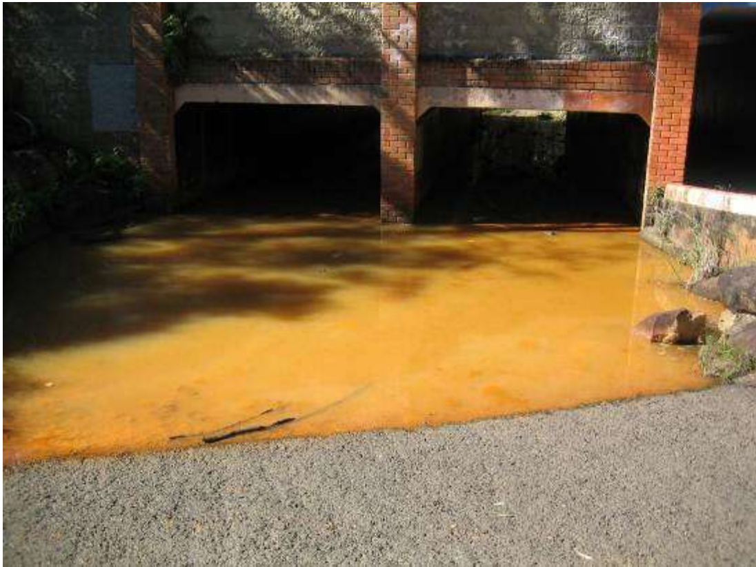
Figure 3-28: Iron (Fe) floc in the tributary to Blunder Creek upstream of the water quality logger, June 2012.
